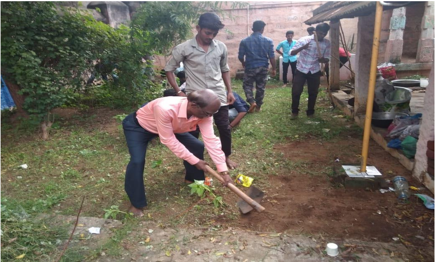
Removal of Glass Bottles and shrubs inside the temple
